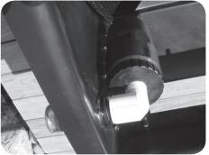
Note: If any leaks are detected locate the fitting, sbut the feed line off and re-tape the beaky fitting. Using a little more tape will usually solve froblem.
