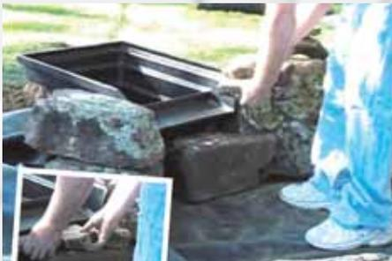
Stack stones up the front of the falls filter to conceal the filter box and liner. Additional stone can be added on top, just below the lip, to extend the waterfall.
