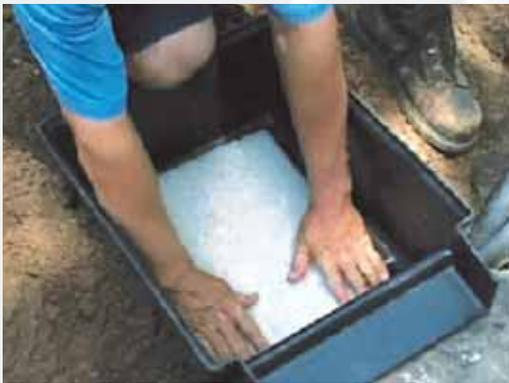
Lay the filter mats in the bottom of the filter box on top of the support tubes or support stands depending on model.
