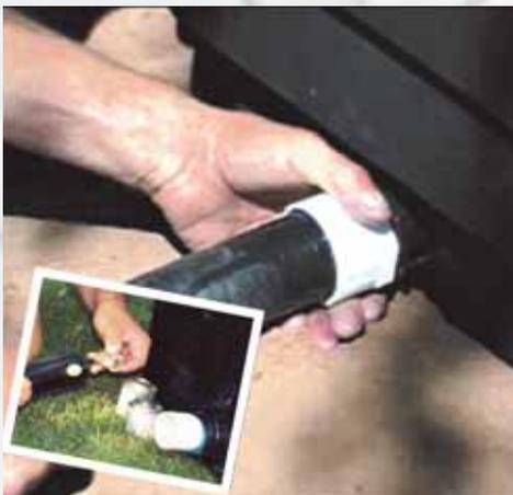
Glue the PVC flex pipe into the male adapter and hold together until glue is set.
