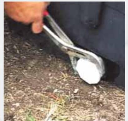
Thread the 2" plug into the unused port using teflon tape or silicone on the threads.
